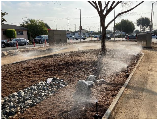
800-2.4 Sprinkler Equipment (Materials) & 801-5.7.3 Irrigation Coverage Test (Installation)
