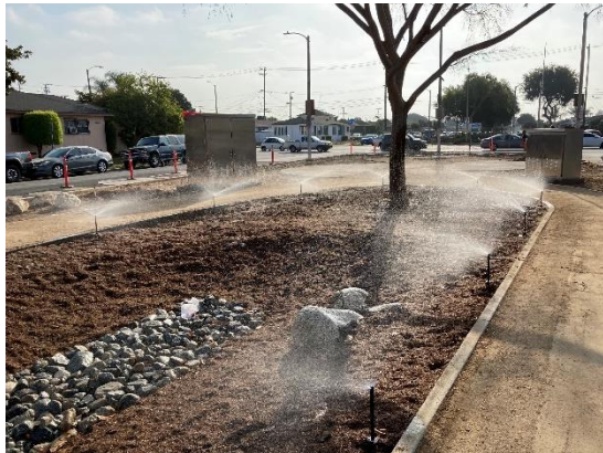
Photos shows: 800-2.4 Sprinkler Equipment (Materials) & 801-5.7.3 Irrigation Coverage Test (Installation)
