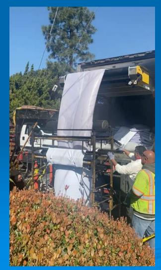
Built in large diameter pipe liner material handling system.
