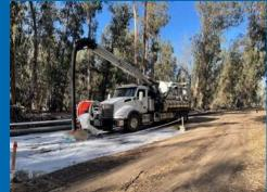
Work area covered, MH sealed around hose and vacuum. Jet hose wash down system
