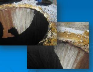
Corroded Concrete Behind Lining System
