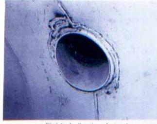
Finished Service Lateral (Cut Flush and Welded)
