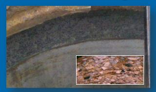
Manhole raised using concrete risers will deteriorate
