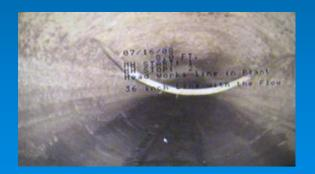
Failing Pipe O-Ring Joints
