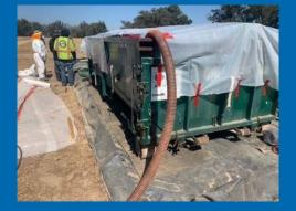
All liquids were filtered in roll off 100 micron filter
