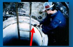
Grout Installation 5,000 PSI Concrete
