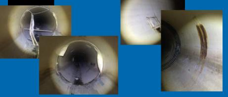
Failing 60 inch T-Lock Pipe Liner joints- 5 miles
