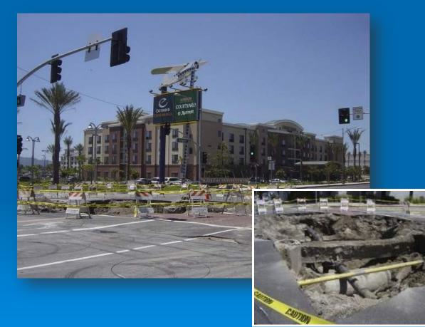
Water Main & Sewer Breaks = Collateral Damage to Other Utilities and the Roads Above
