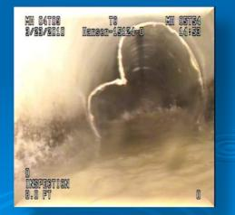
Failed CIPP Spot Repair installations Ambient Cure Resins
