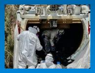
Debris tanks were hand cleaned and bagged by certified asbestos crews
