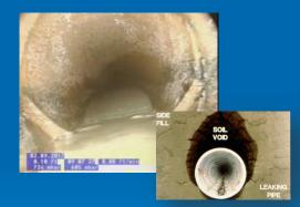
Infiltration Pipe backfill washing inside the pipe
