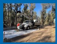
Work area covered, MH sealed around hose and vacuum. Jet hose wash down system
