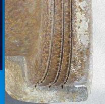
Bottom of pipe joint No mortar
