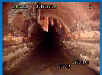
Sheets of Asbestos pealing off
