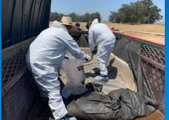
Debris in 100 micron tank filter were cleaned and bagged by asbestos crews
