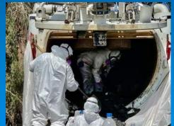
Debris tanks were hand cleaned and bagged by certified asbestos crews
