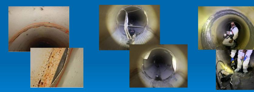
120" Inner Plant Pipeline Failed PVC Joint Welds 60" Trunk Pipeline Failed PVC Joint Welds Transition from 60 inch CIPP Liner to New PVC Pipe
