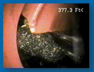
Blacktop Paving or Rocks used in Backfill
